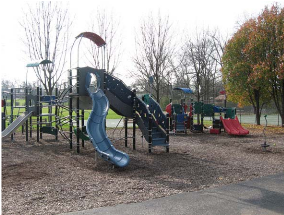
Photo 9: EWF noted with observed undulating surface.
