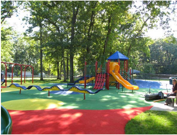
Photo 13: HYB surface system designed with outdoor carpet as top layer over engineered carpet pad base and infilled with silicone sand.
