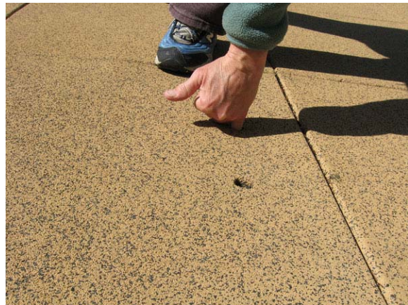
Photo 8: TIL with puncture holes.
